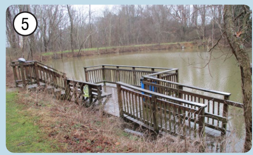
EXISTING CONDITION FIVE
