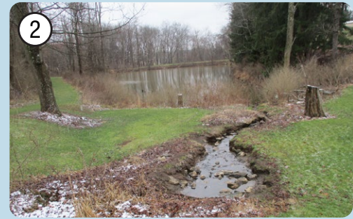
EXISTING CONDITION TWO
